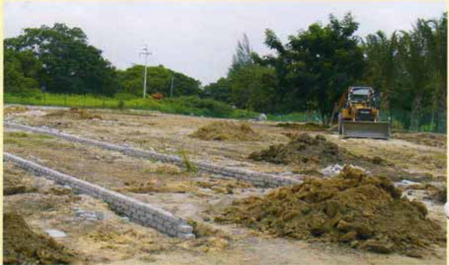
▲ Levelling of the ground.
