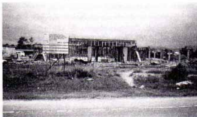
New Building under construction
